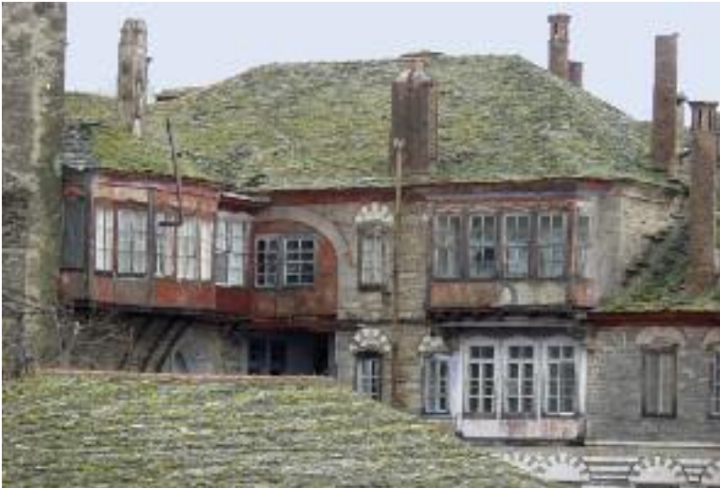
Part of the South-West Wing, which has not been renovated.
