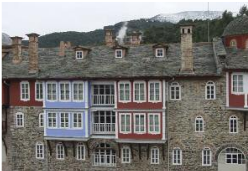
The East Wing after restoration.
