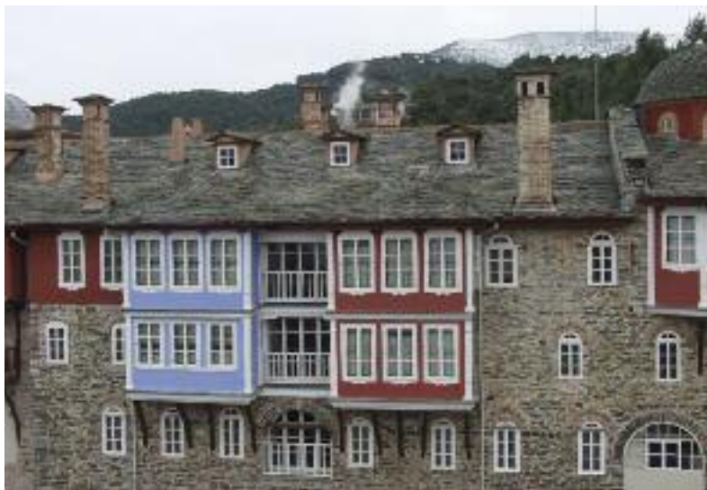
The East Wing after restoration.
